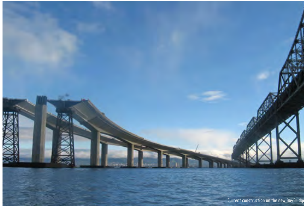
Current construction on the new Bay Bridge
