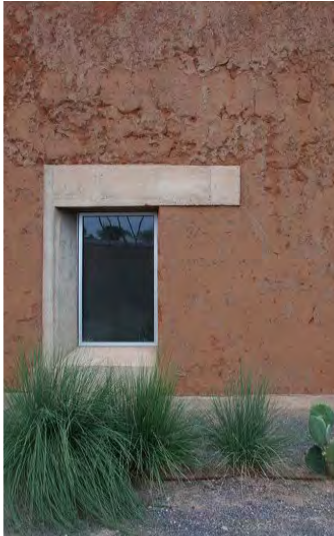
Two types of mud bricks, or adobes, were used in the construction. The lower portion has adobes made in New Mexico that possess a higher compressive strength and resistance to water. Towards the top of the wall, adobes made in nearby Ojinaga, Mexico were used that are lighter in both weight and color. The mud used in the plaster is from Van Horn and has a beautiful reddish tint.
