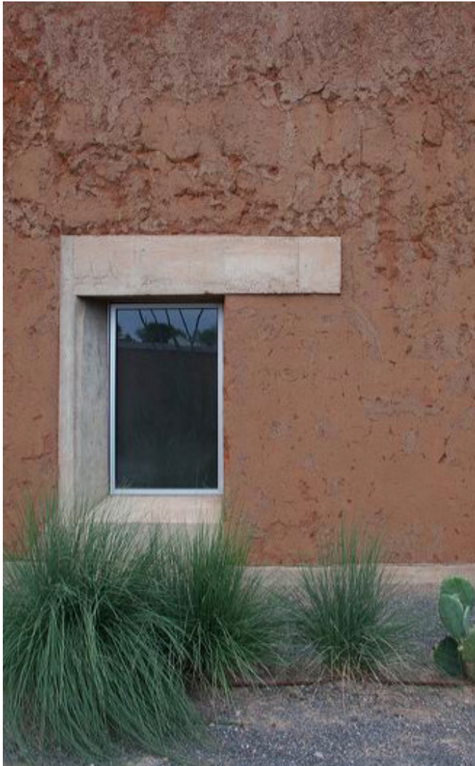
Two types of mud bricks, or adobes, were used in the construction. The lower portion has adobes made in New Mexico that possess a higher compressive strength and resistance to water. Towards the top of the wall, adobes made in nearby Ojinaga, Mexico were used that are lighter in both weight and color. The mud used in the plaster is from Van Horn and has a beautiful reddish tint.
