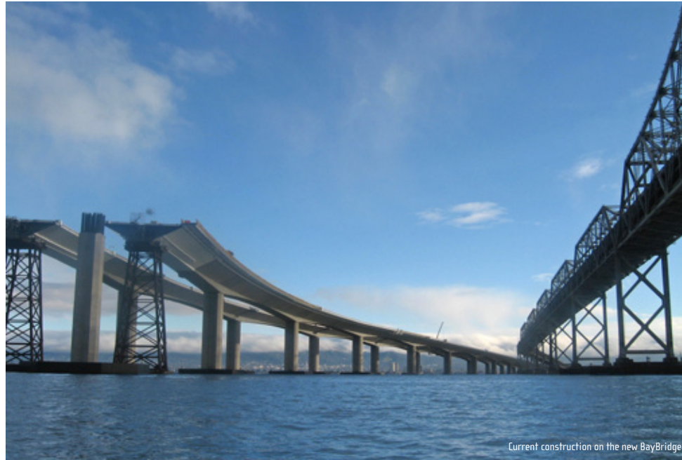
Current construction on the new Bay Bridge
