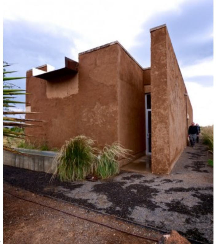
right: north wall with scupper
