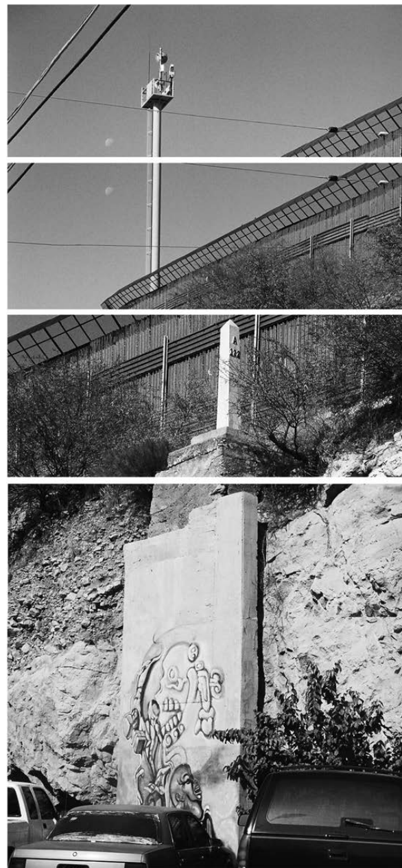
Monument 122-A, viewed from the Avenida Internacional in Nogales, Sonora. A fortuitous vertical stacking of boundary infrastructure recalls the deep archeology of the line. The top panel reveals present-day electronic surveillance apparatus; below this is the 1990-era Operation Hold-the-Line fencing (made from recycled aircraft landing mats from the Vietnam War); in the third horizon is a monument from the late-nineteenth-century boundary resurvey; and at its base lies a concrete retaining wall that has been spray-painted with symbols of birth and death characteristic of ancient Mesoamerican cultures.
