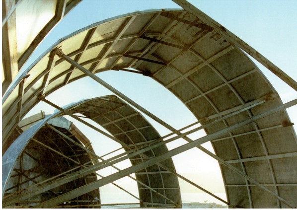
FIG. 9 : METAL FORM WORK FOR ICE HOTEL
