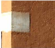
concrete lintel above bedroom window
